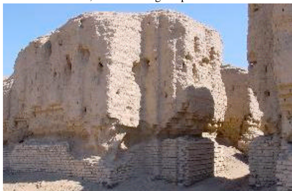
Similar walls, once uncovered show how the sand had protected the lower layers of brick.
