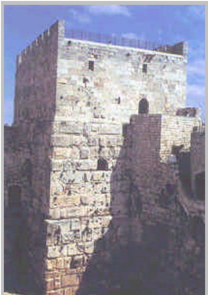
Known as the 'Tower of David', this portion of the Citadel was actually constructed by Herod with the top portion being added as a repair by the Crusaders.
