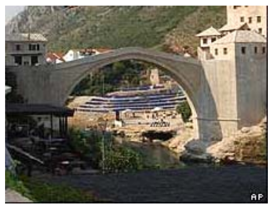
The reconstructed bridge
