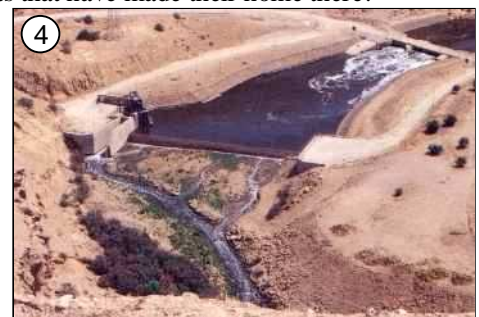
④ Below Peniel, salt springs make the water unsuitable for irrigation. This weir diverts most of the Zarqa river water before it becomes saline.
